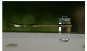
This shows how the side hook is fixed. The nut between the plastic and the hook puts it in the right position to hook over the bolt.
