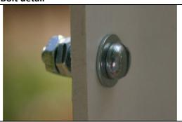
The bolt sticks out to the side so that the hook can fasten over it. There is one nut, then a space, then two more nuts. The hook goes round the space.
